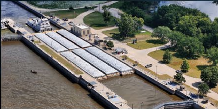
Lock and Dam 13 on the Mississippi river at Fulton, IL loading the lock so a barge can proceed down river.
